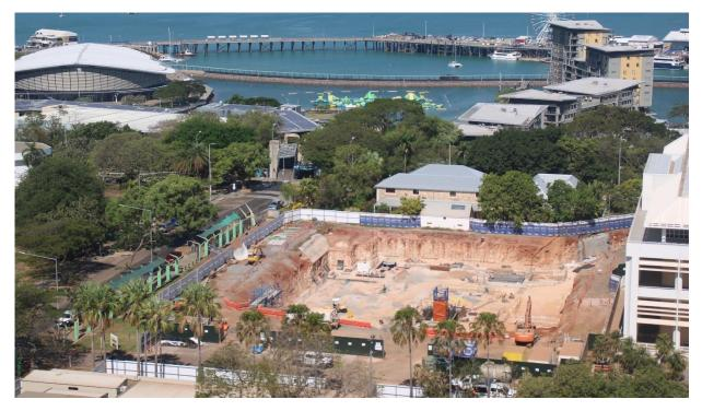
Construction of the Northern Territory Art Gallery is at the basement level after in-ground services, including plumbing, were completed in July 2023.
